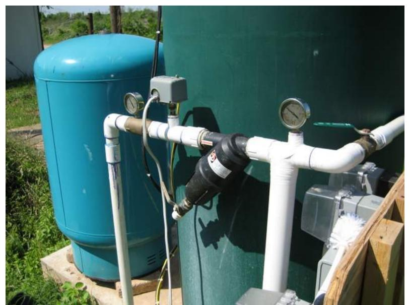
After the water has passed through these filters there are two different directions it can take – either it will go to the houses or it will go to the fields. Water that goes to the houses goes through a booster pump and a pressure tank located at the well. Water for the fields is directed to the barn where there is another booster pump and two large black storage tanks totaling 5,500 gallons.
